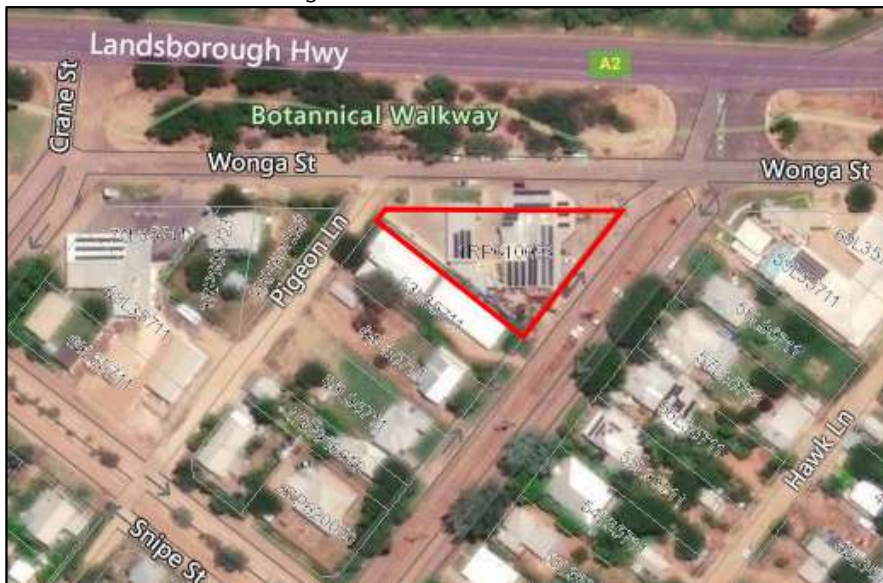
Figure 1 – Subject site and locality (Queensland Government DAMS)
