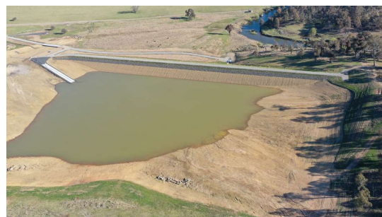
Walcha off-stream storage dam built as part of the NSW Connections Package. Photo courtesy of Walcha Council.
