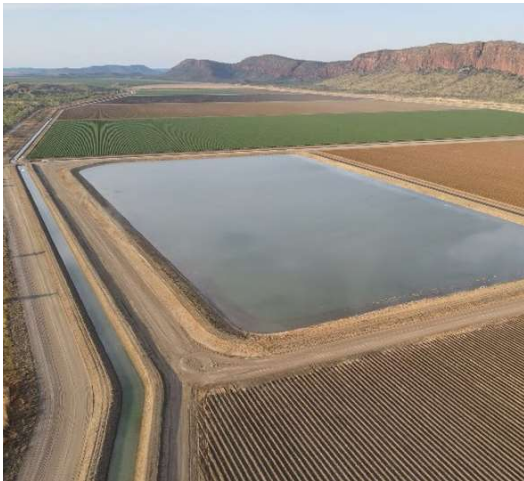
Cave Springs Road Tail Water Return System, part of the Western Australia Connections package. Photo courtesy of the Western Australian Government.
