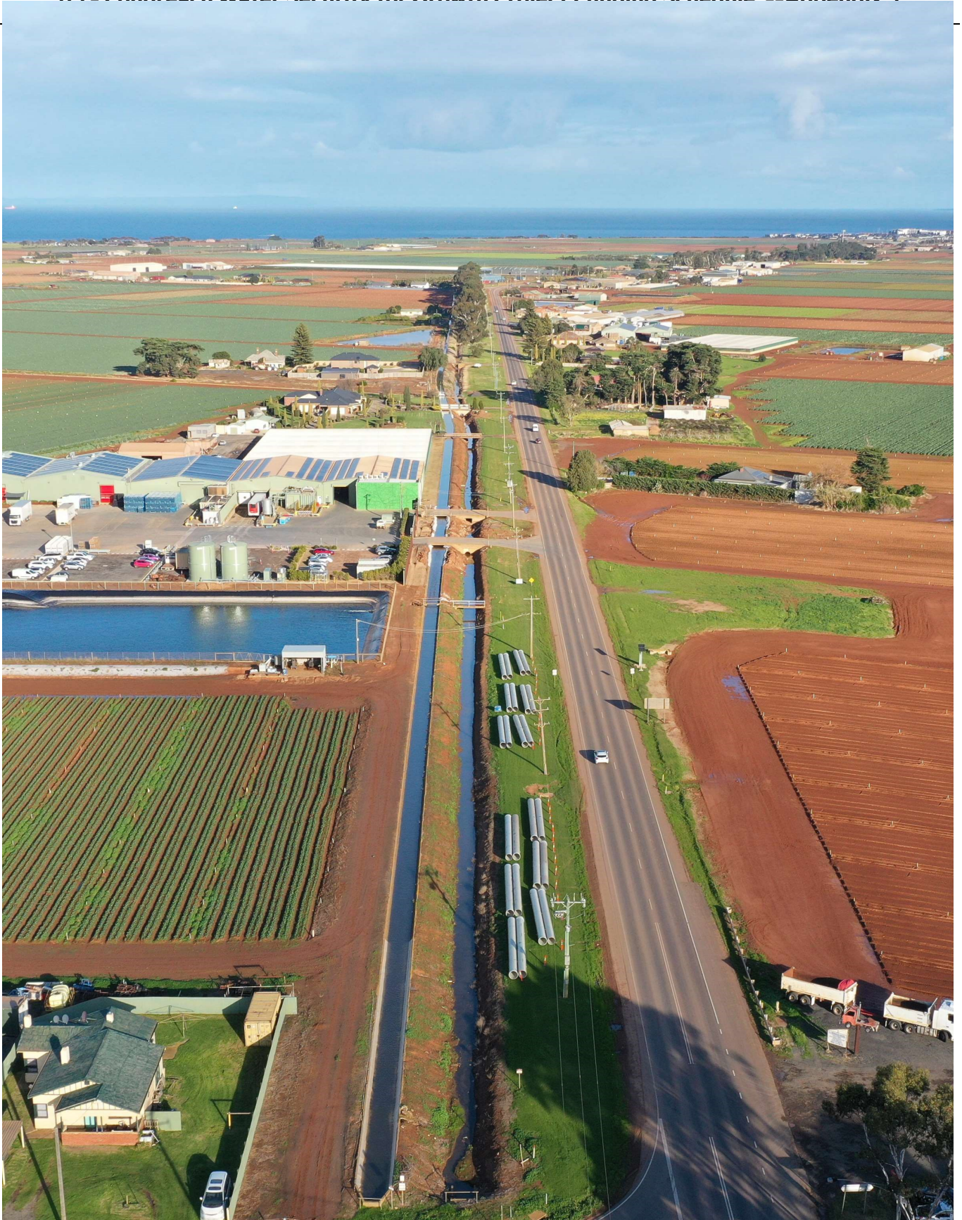
Werribee Irrigation District Modernisation project, Victoria. Photo courtesy of Southern Rural Water.
