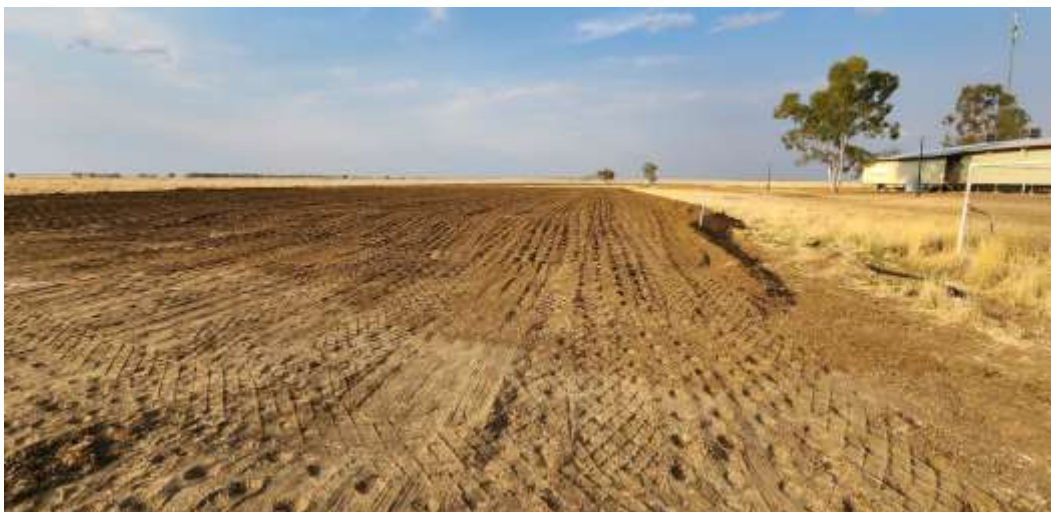
Ilfracombe Multi-sport court site preparation
