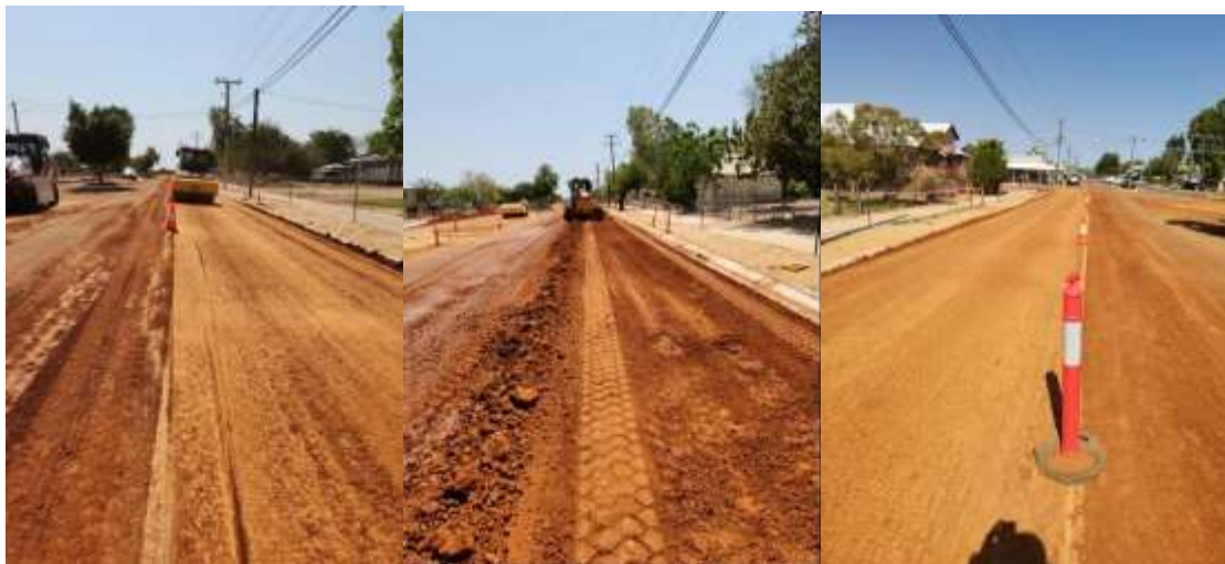
Saint Mary Street Isisford – new curb installation and rehabilitation project
