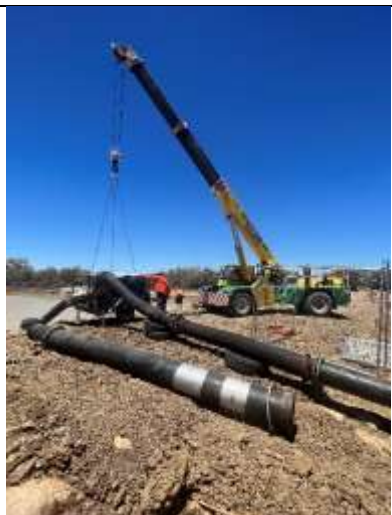
Relocating the pump at Fairmount Weir to increase pumping performance.
