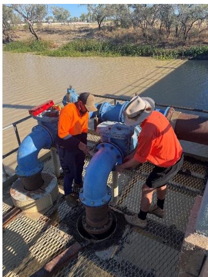
Plumbing crew carrying out maintenance works to the raw water pumps at Thomson River.
