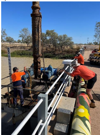
Plumbing crew carrying out maintenance works to the raw water pumps at Thomson River.
