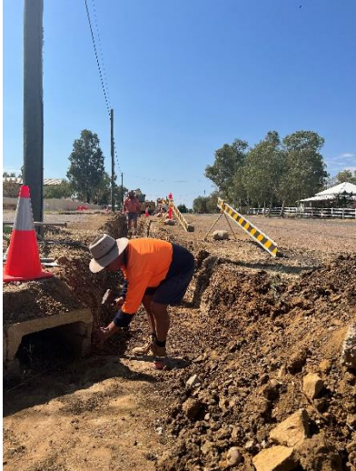
Culvert replacement at Wellshot Street Ilfracombe.
