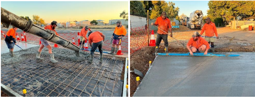
Corella Lane – drainage slab installation.
