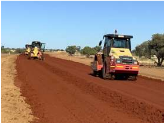
Treatment of base course on the Stonehenge River Road project.
