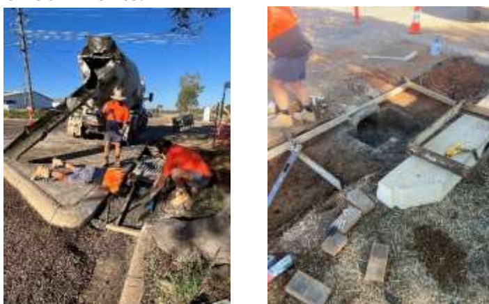
Upgrades to stormwater network in Longreach Streets.
