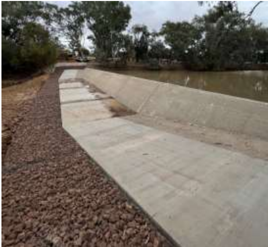
Isisford Weir completed at the Barcoo River.
