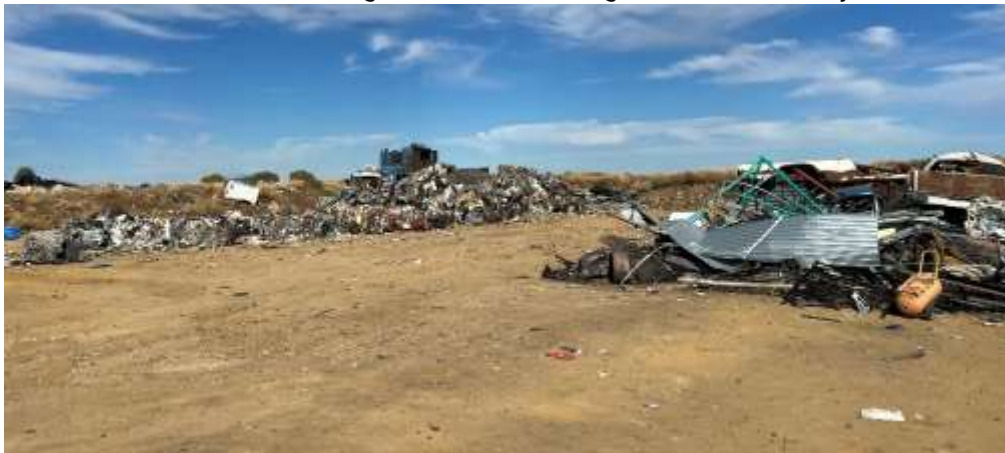
Removal of scrap metal waste at Longreach
