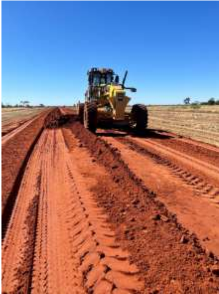
Sub grade on Longreach-Jundah Road rehab.
