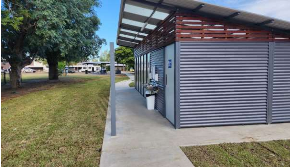
New Edkins Park Toilet Block
