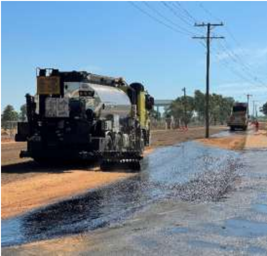
Longreach Construction Crew conducting seal of Kite Street.
