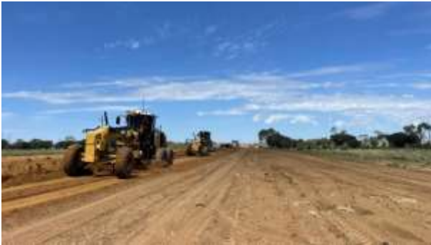
Ilfracombe Construction Crew – Jundah Road rehab job.
