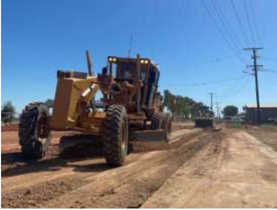
Longreach Construction Crew working on Kite Street widen and seal.
