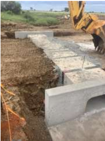
Culvert replacement on Stonehenge River Rd.
