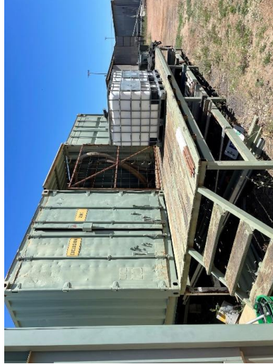
Photo 5: Depot - Fall risks at Exclusion containers
