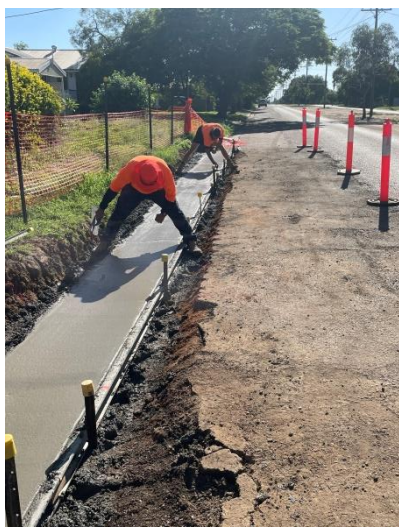
Gutter repairs in Wompoo Road completed by the Concreting Crew.
