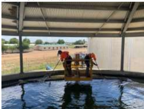
Cleaning of clarifier launder trays – Longreach WTP
