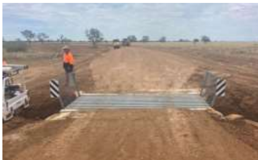
RMPC Grid Relocation – Longreach Jundah Road to the Notus Downs Road
