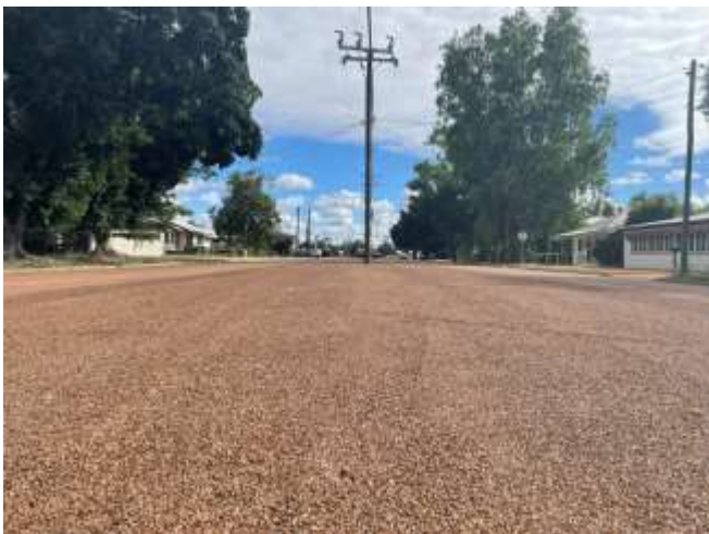
Centre sealing of Cassowary Street between Wonga & Snipe Street - completed
