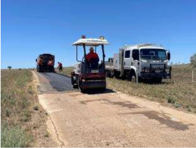
Sealed Network Team Reseal prep – Morella Silsoe Road.
