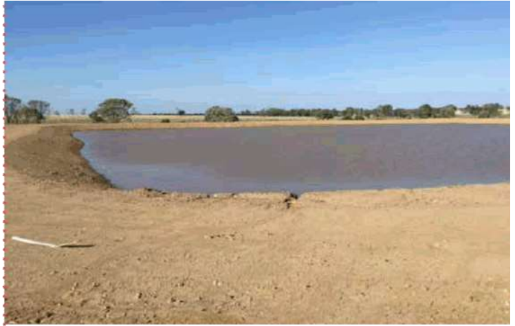
Nogo Water Facility
