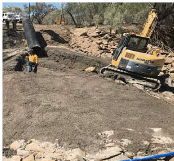
Longreach Weir Repairs (Thomson River)
