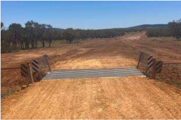
New Grid Installation completed – Morella Silsoe Road.
