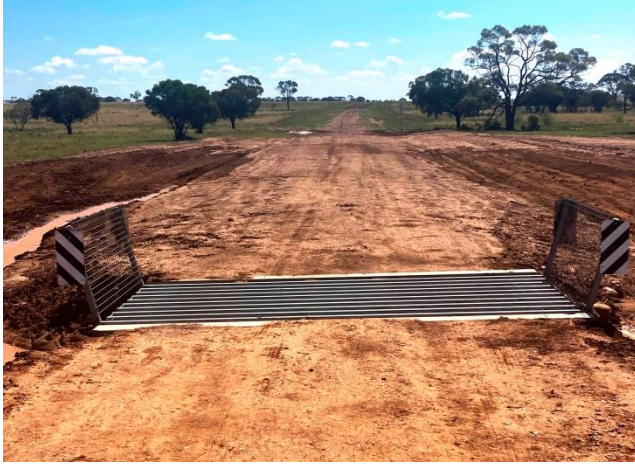
New Grid Installation completed – Bogewong Alroy Road.
