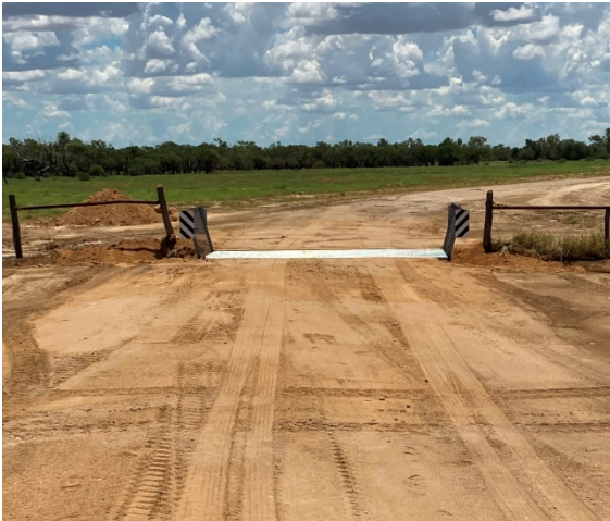
Grid Replacement on Darr River Downs Road during 2020/2021.
