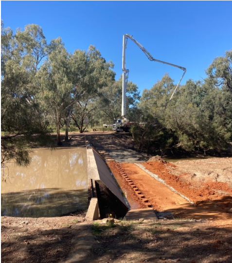
Isisford Weir Upgrade – Pump Truck ready to pour.
